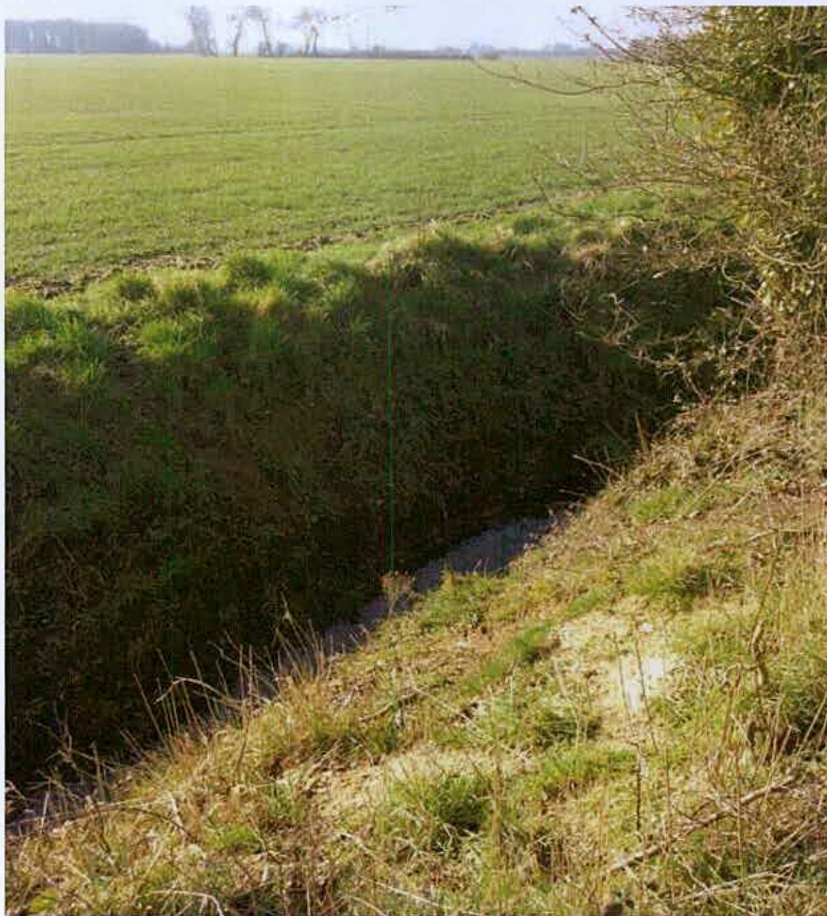
Figure 7. The wet ditch running along the southern boundary of the site.
