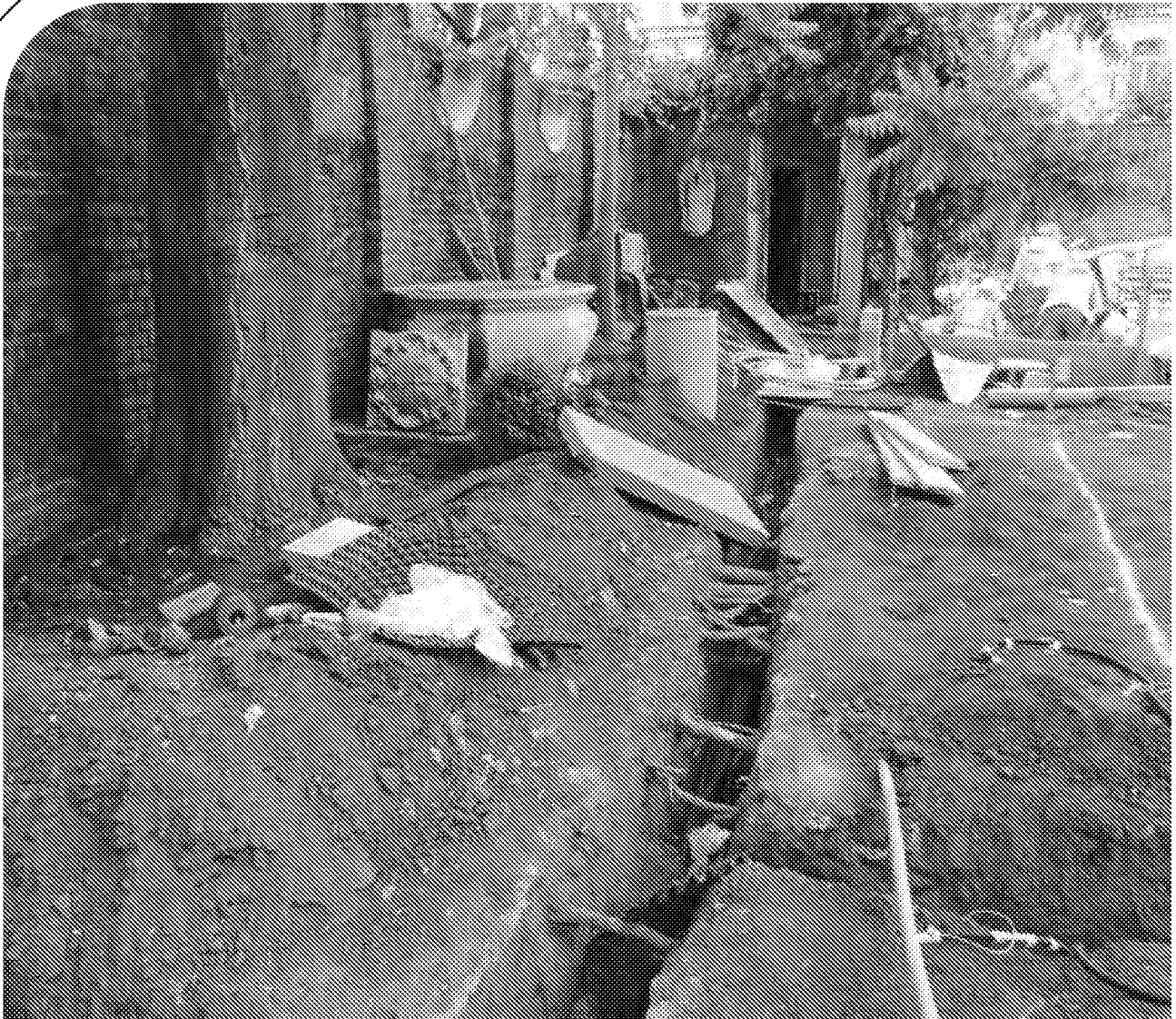
Site Guidance Note 7: Excavation in root protection areas
