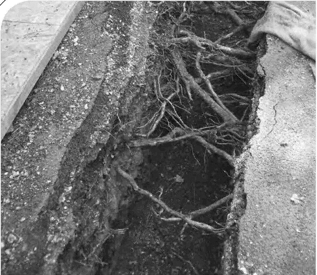
Site Guidance Note 8: Removing surfacing and structures in root protection areas
