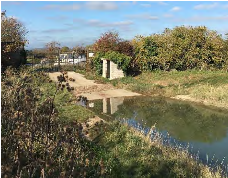
Image 2.16: Obstruction of Footpath 206
