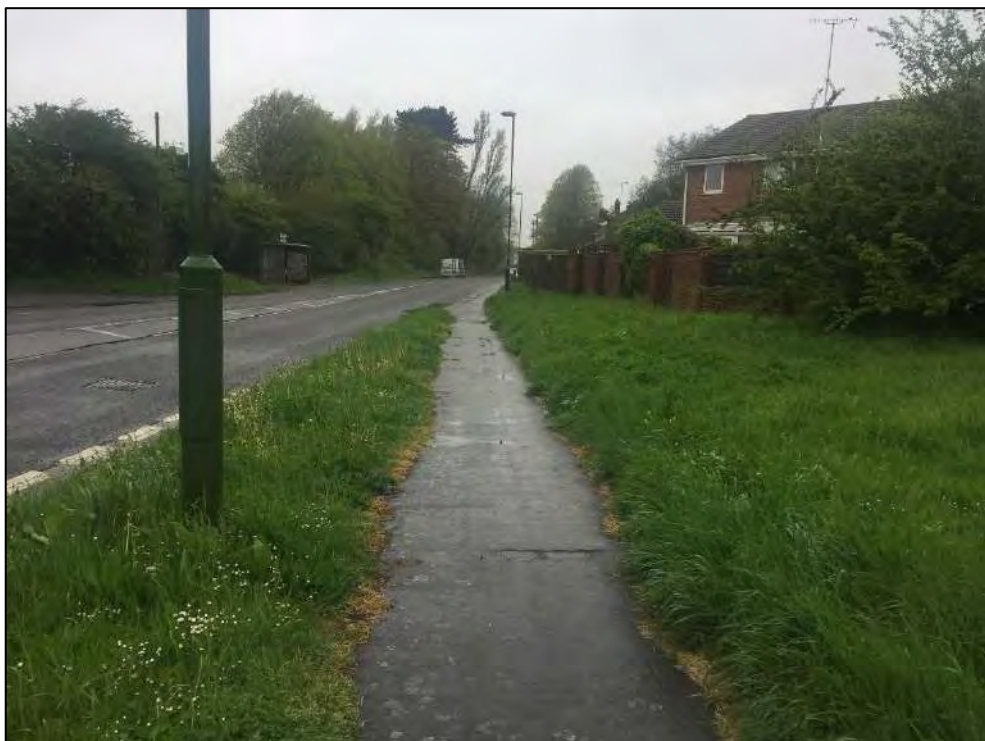
Image 2.6: Footway provision from Rollaston Park Road along Yapton Road heading north west
