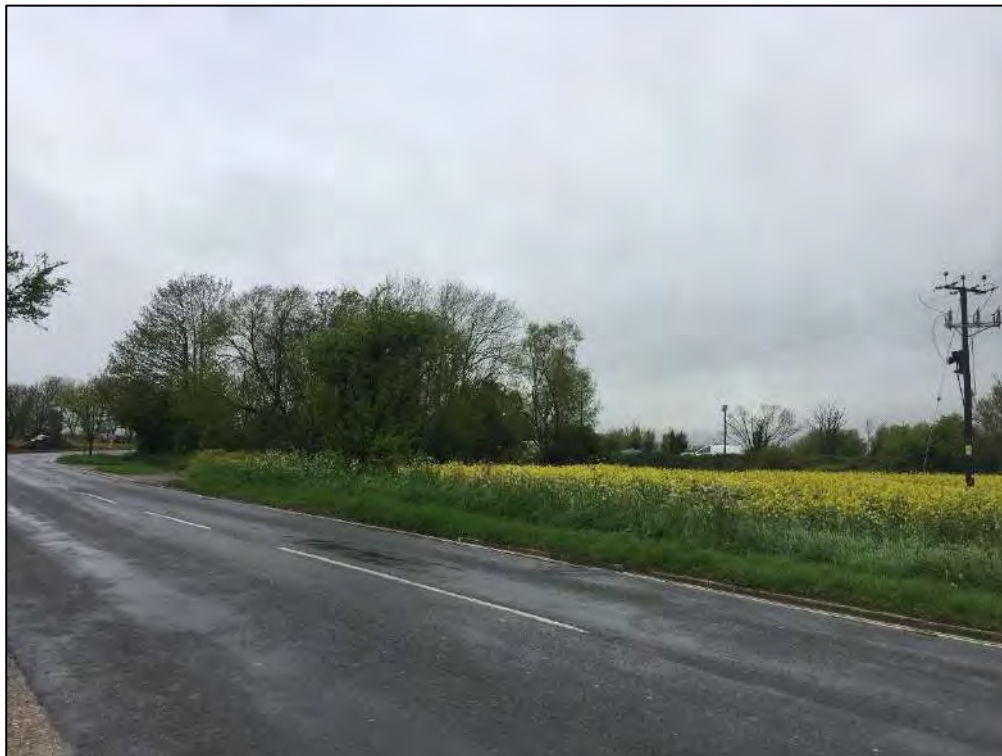
Image 2.9: Footway provision along Ferry Road
