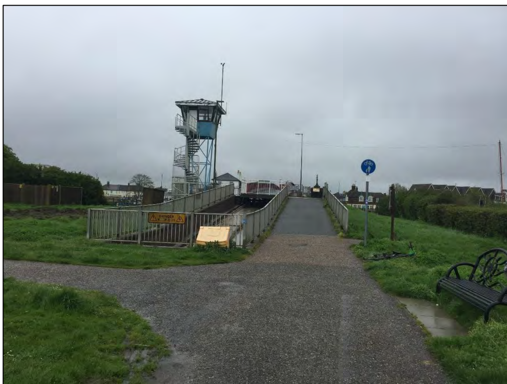
Image 2.10: Footbridge over the River Arun to Littlehampton
