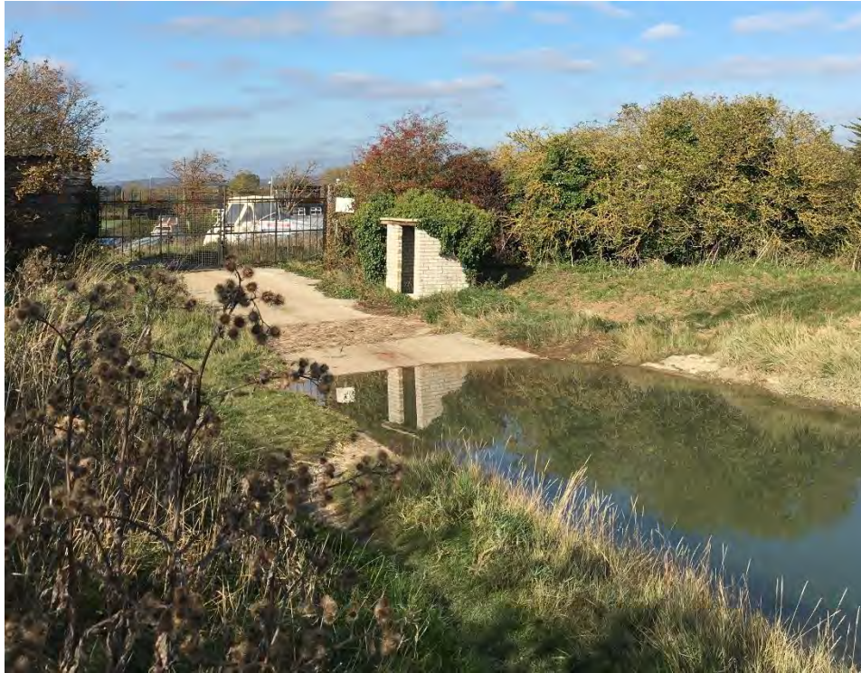
Image 2.16: Obstruction of Footpath 206
