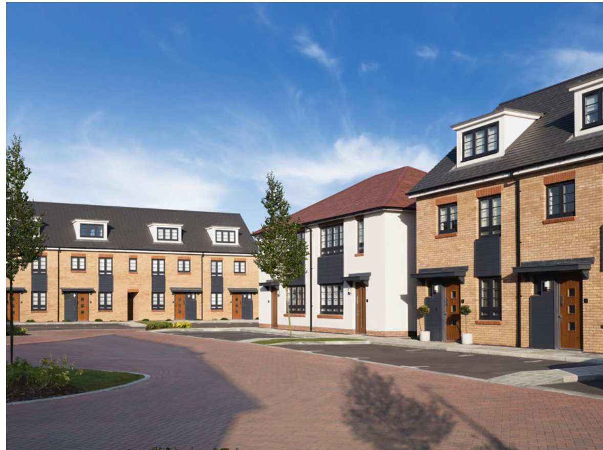
Figure 177: Good quality surfacing materials and planting contribute to soften the streetscape
