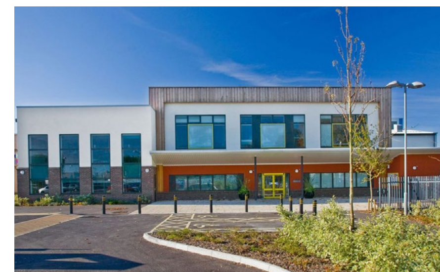
Figure 166: Local Precedent: Southway Primary School
