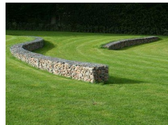
Figure 101: Gabion walls using recycled concrete providing structure in parkland
