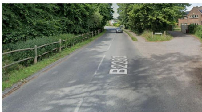
Burndell Road Looking Northwest
