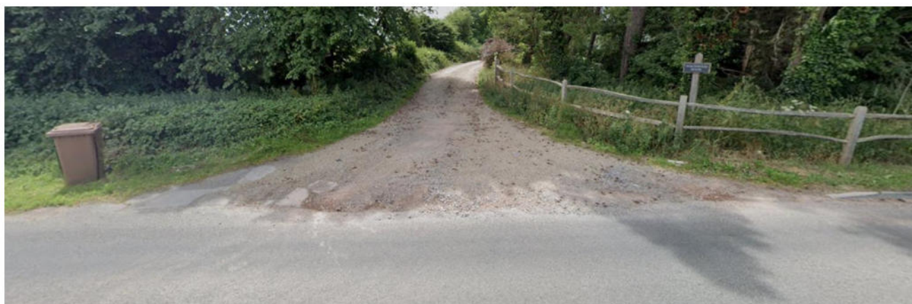
Figure 2.2: Existing Access Point
