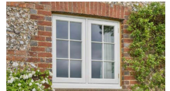
Painted Timber Casement Windows
