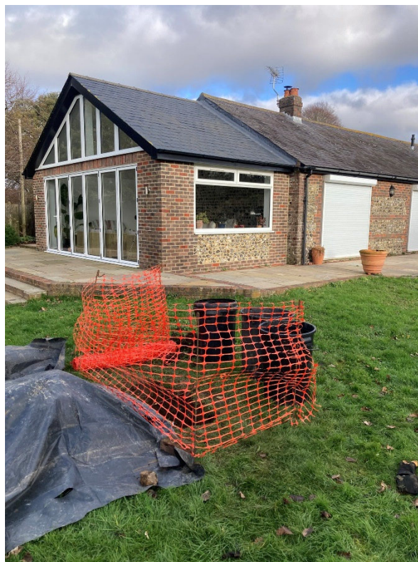
Photograph 7 : Trial Pit TP4 Location
