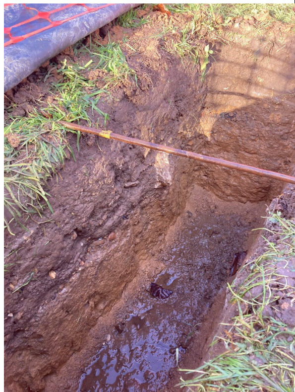
Photograph 8 : Trial Pit TP4 after test
