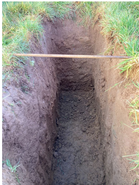
Photograph 6 : Trial Pit TP3
