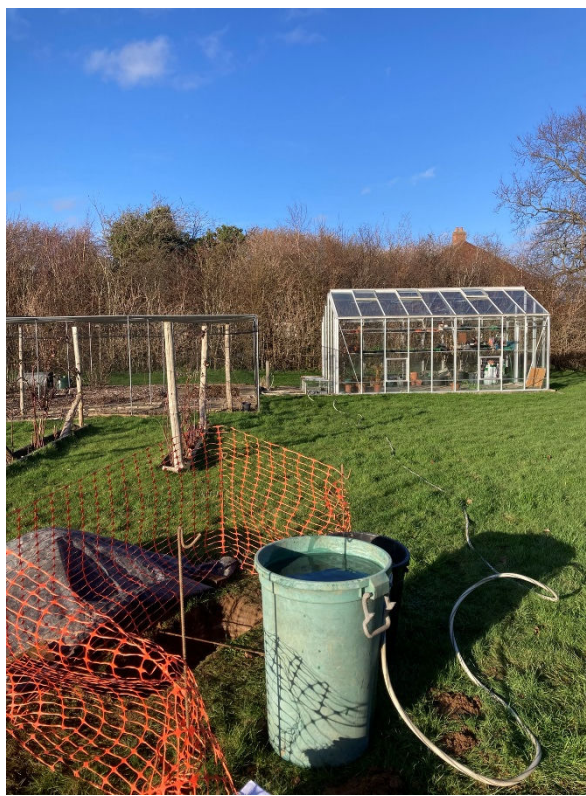
Photograph 3 : Trial Pit TP2 Location
