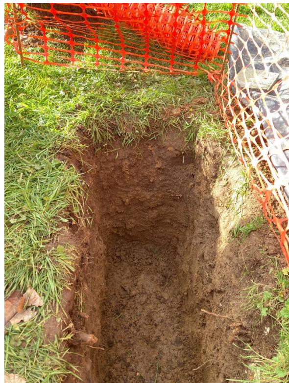
Photograph 2 : Trial Pit TP1
