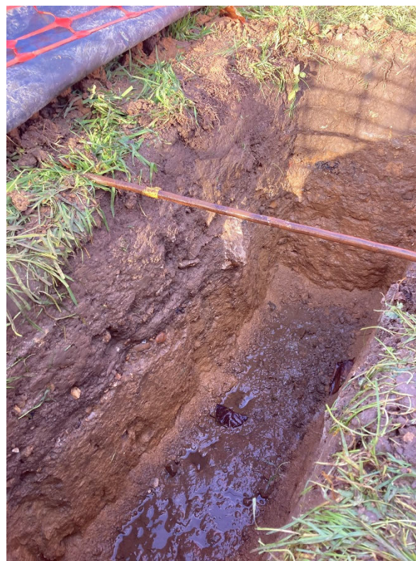
Photograph 8 : Trial Pit TP4 after test
