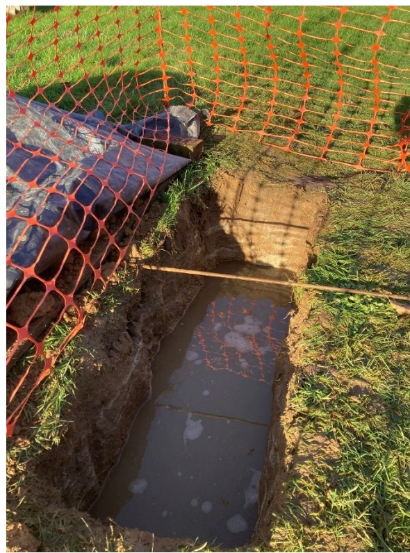
Photograph 4 : Trial Pit TP2 under test
