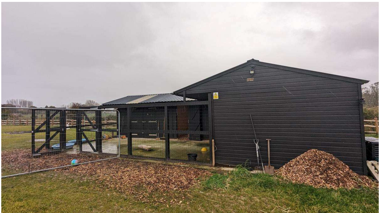
Photo 4 – View of the building on site looking west.
