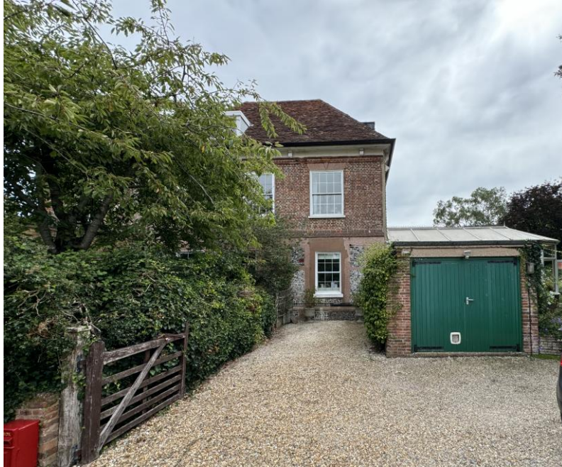
West Elevation, including conservatory roof visible beyond modern single storey flat roofed store room (former garage)
