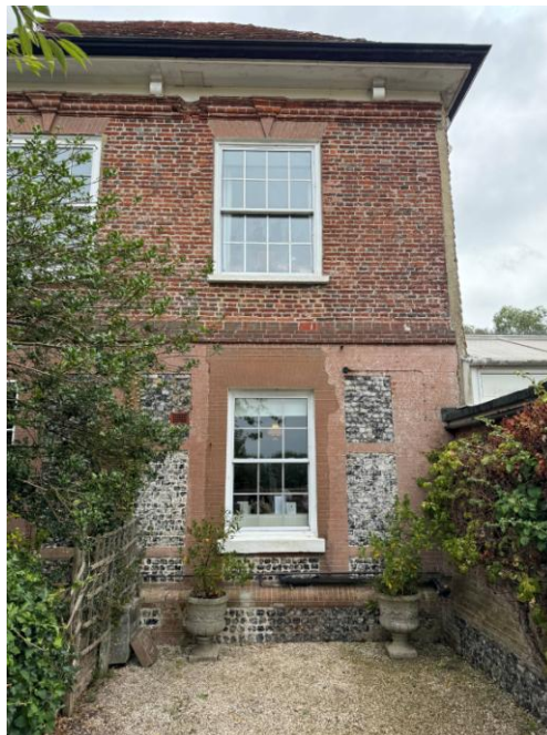
Detail of West Elevation, showing the section of Atherington House which formed part of the original property, 'Ford Place' and works recently undertaken to the walling surrounding window opening in the 2020s
