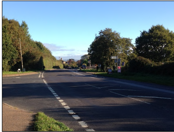
Figure 4. Photograph of the Ford Road / Ford Lane Junction
