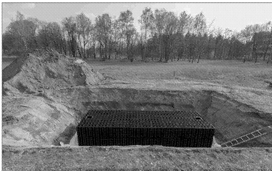
Stormbloc® Optimum installation.
