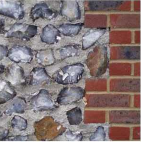
Knapped Flint Blocks with Birdsbeak Pointing Olde Woodford Red Multi brickwork used for detailing
