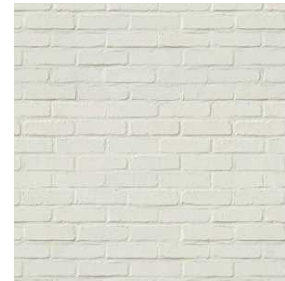
Painted Brickwork Colour - White
