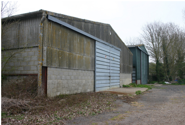
Blockwork and Profiled Steel Storage at New Barn Farms BP Commercial Offices
