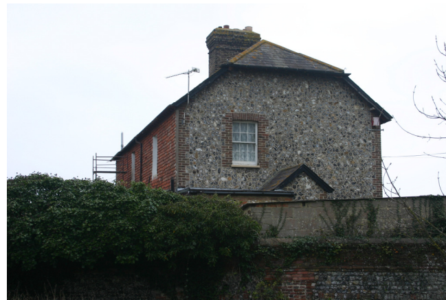
Traditional Knapped Flint Farm Building close to Mill Studio
