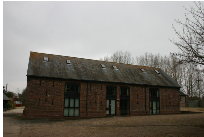
Brick Faced Commercial Offices at New Barn Farm Business Park
