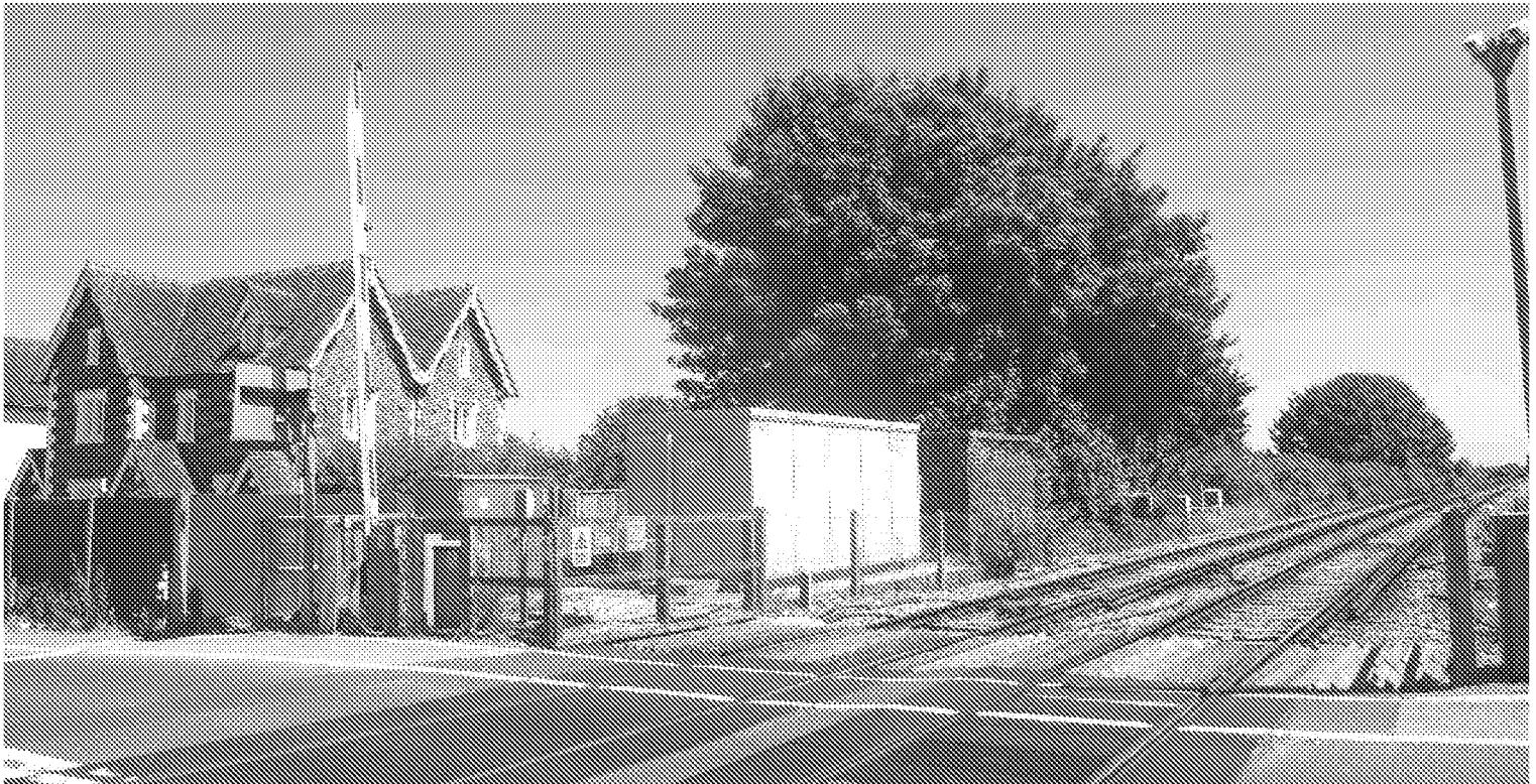
4.4.1 View north east to sycamore clump. Sycamores on right are a long way off-site.
