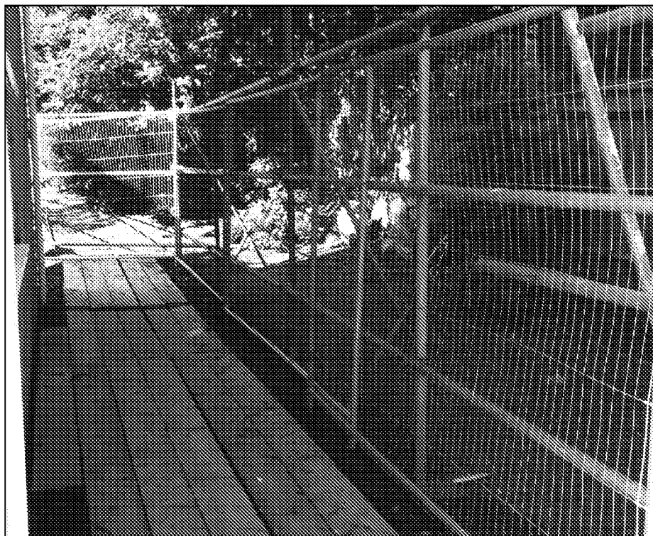
Scaffold board pedestrian ground protection
