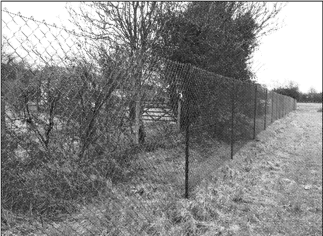
Chain-link on angle-iron uprights
