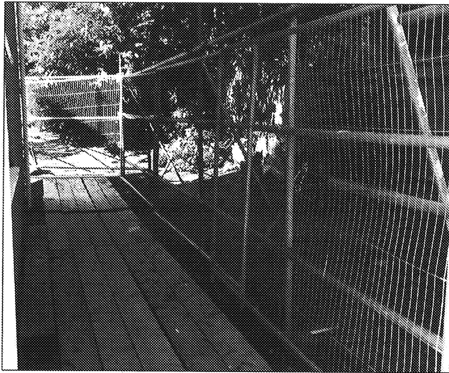
Scaffold board pedestrian ground protection
