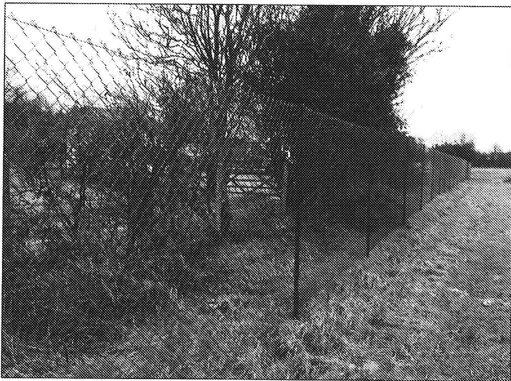
Chain-link on angle-iron uprights
