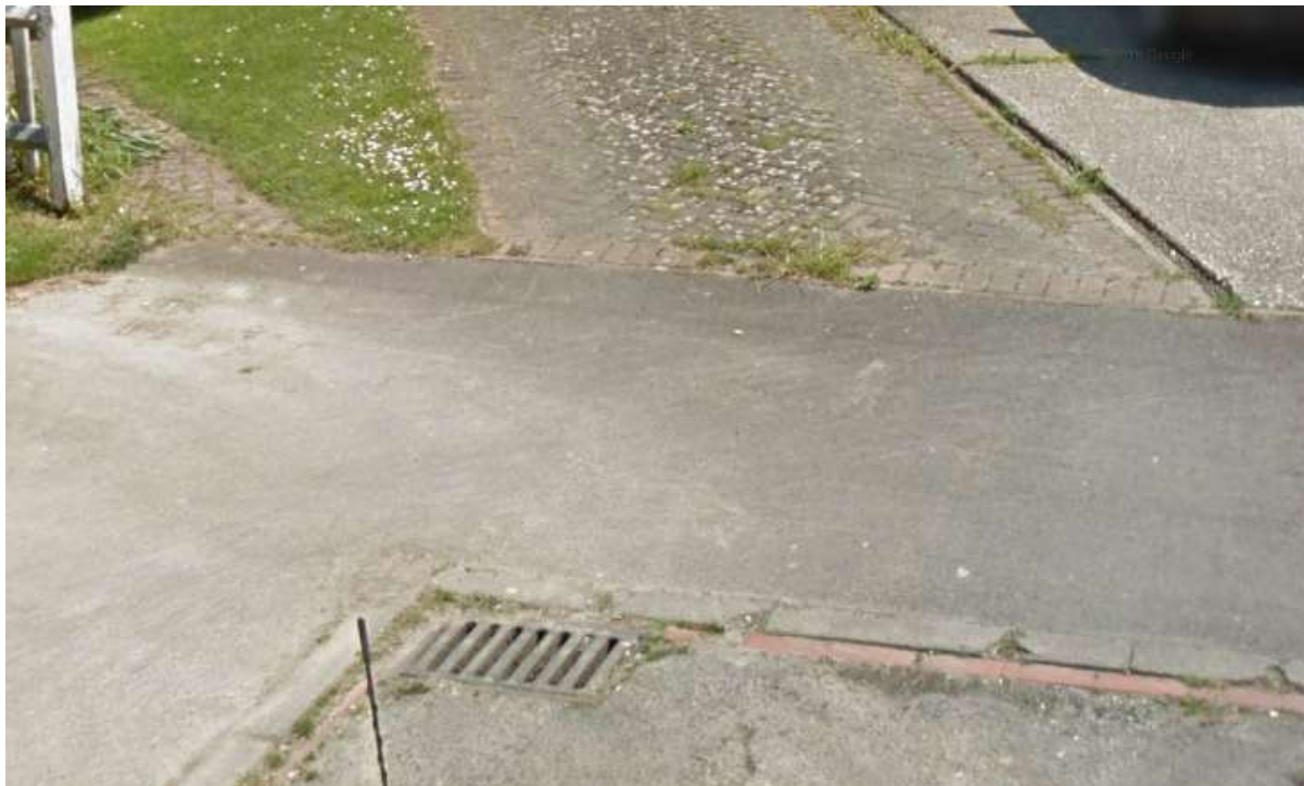
Image 3.2: Existing Dropped Kerb
