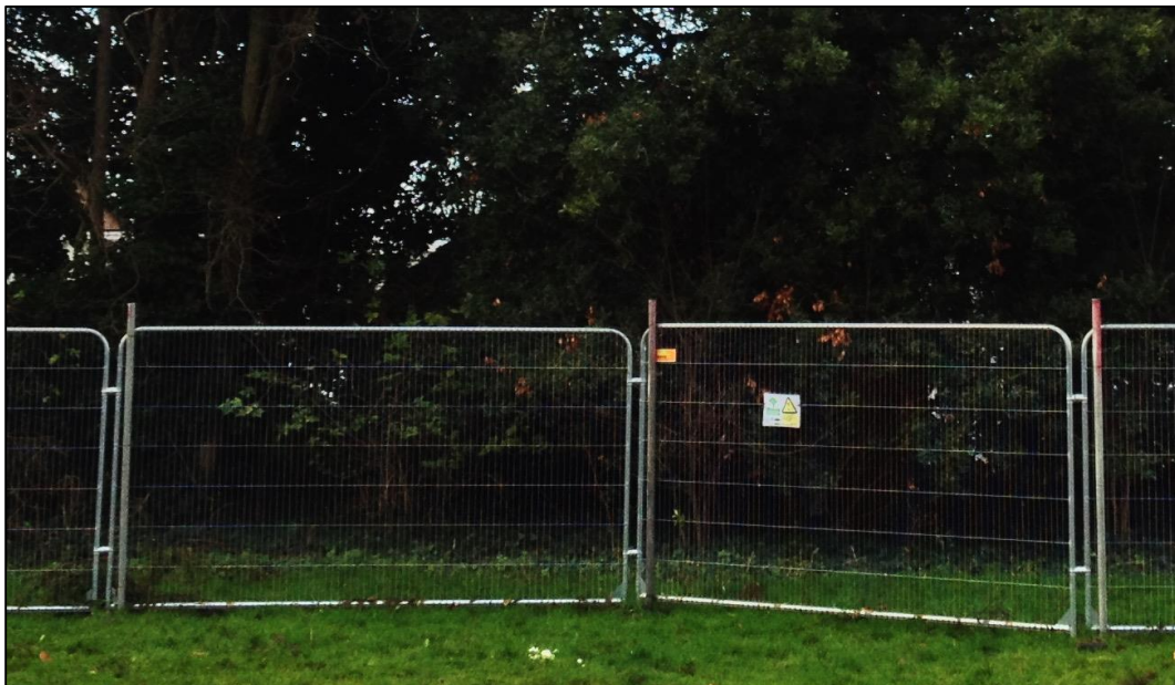
Weld-mesh panels on scaffold uprights
