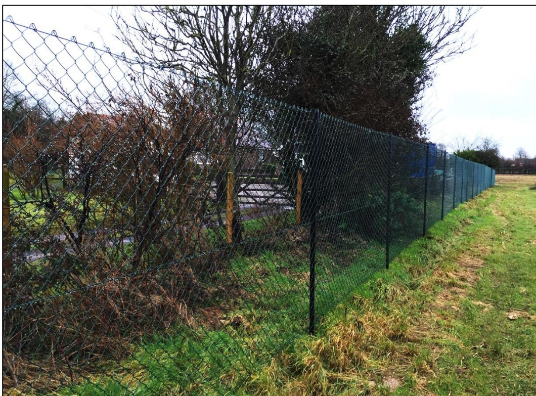
Chain-link on angle-iron uprights
