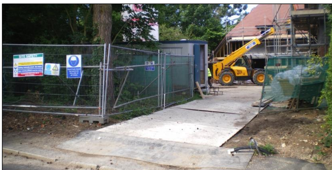
Vehicular ground protection trackway
