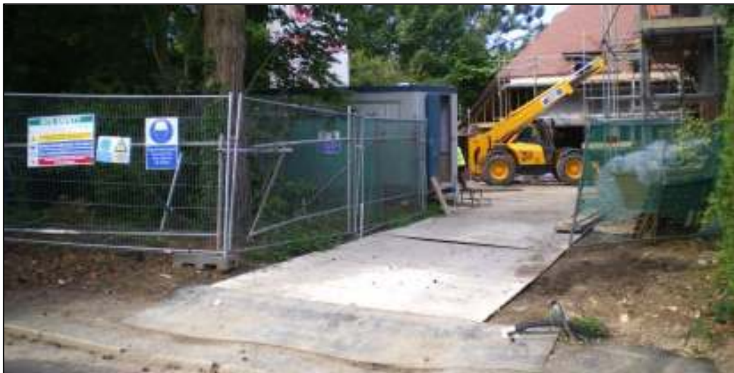
Vehicular ground protection trackway
