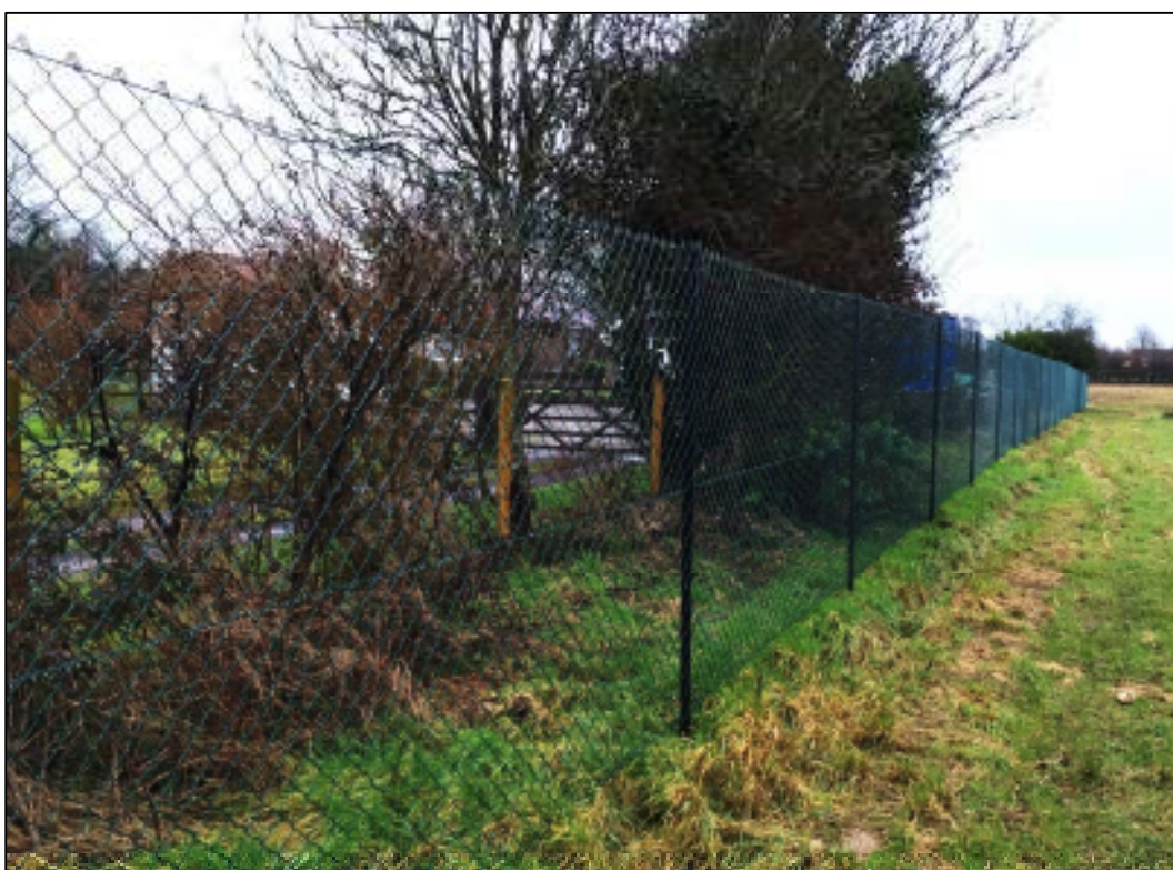
Chain-link on angle-iron uprights
