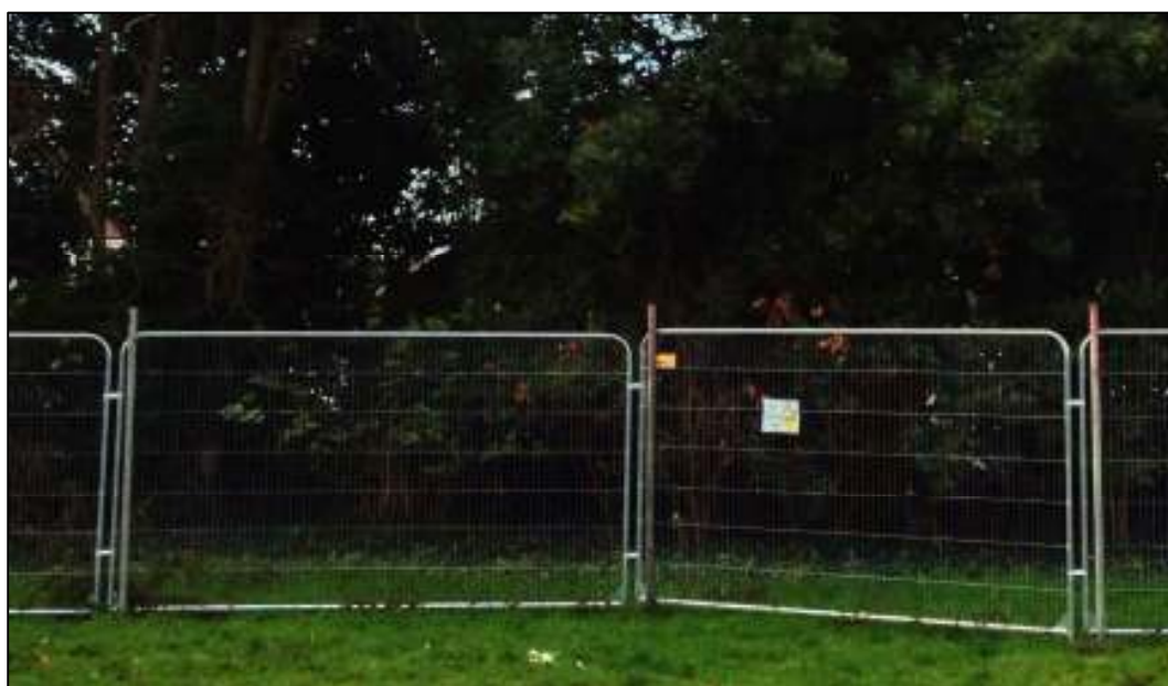
Weld-mesh panels on scaffold uprights
