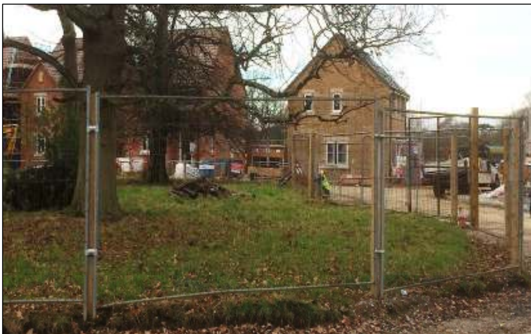
Weld-mesh panels on wooden posts
