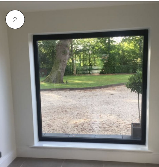
Internal view of window
