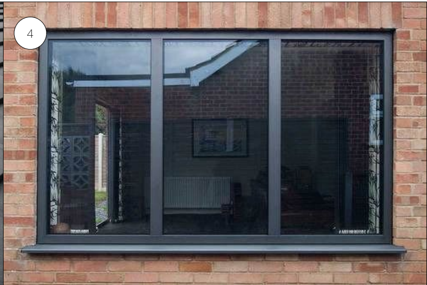
Black powder coated windows - windows to be inserted in to white render on ground floor and cladding on first floor
