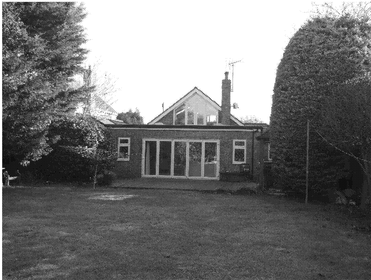
Rear, west facing elevation 57 Downview Road.
