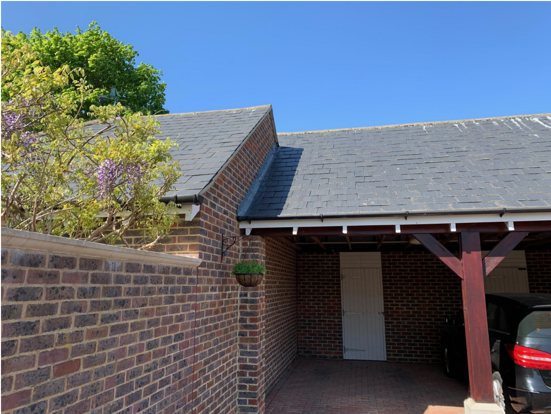
rear (east) elevation - showing relationship to car barn
