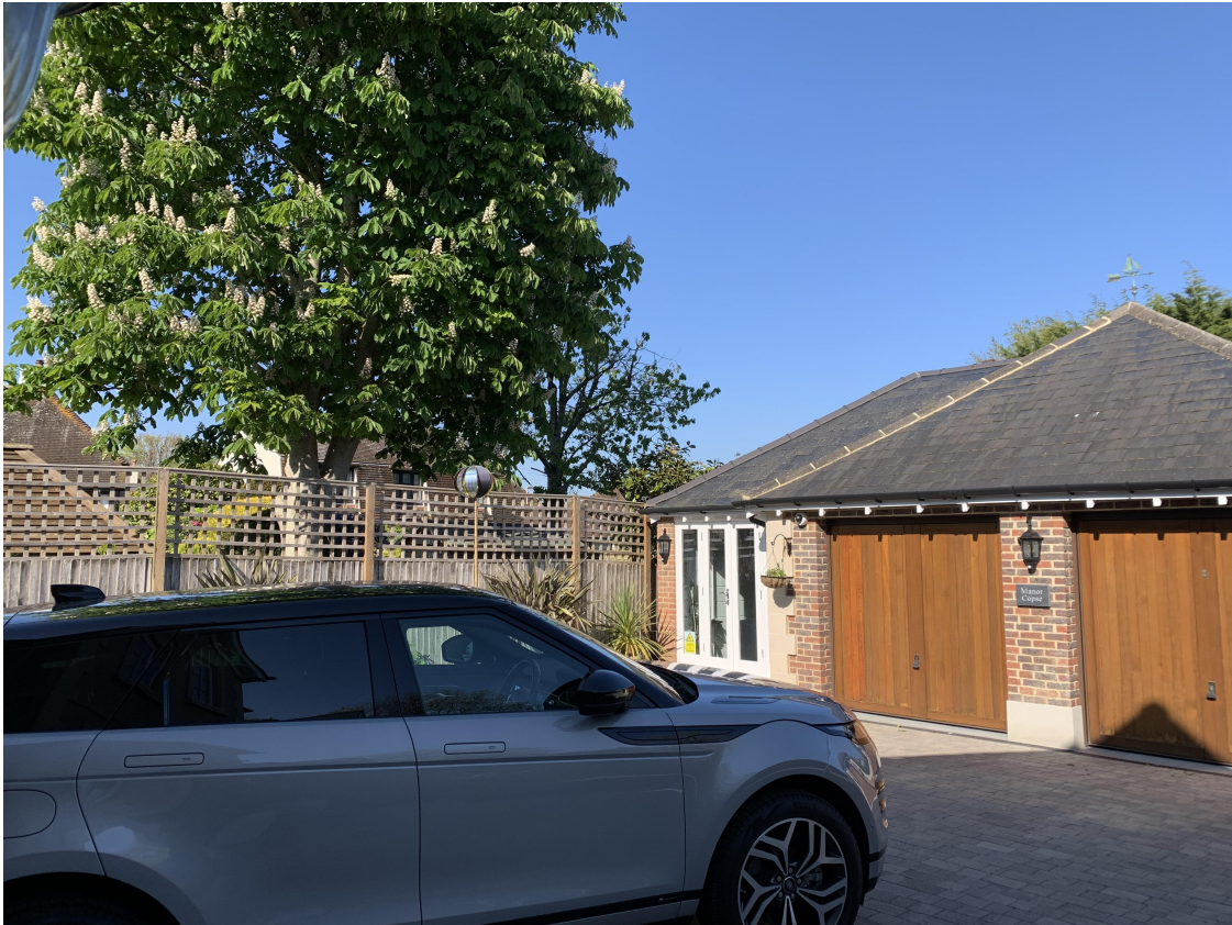
front (west) elevation - showing boundary screening
