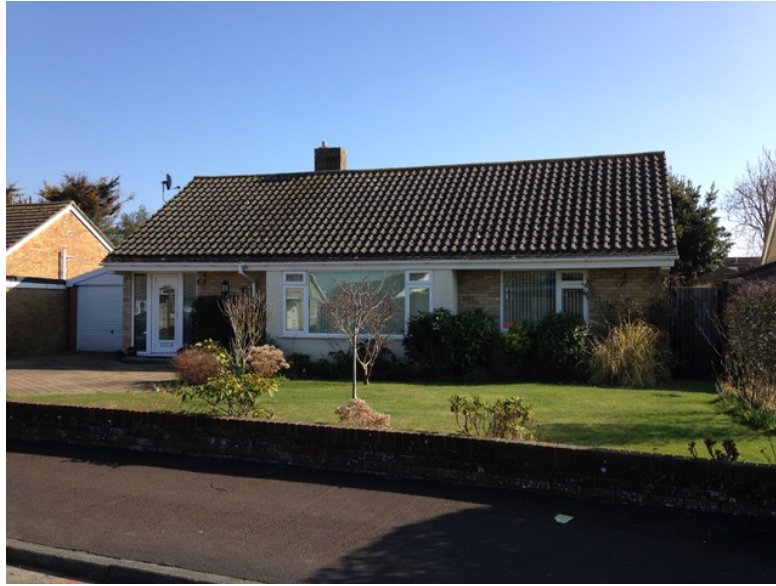
The existing front elevation
