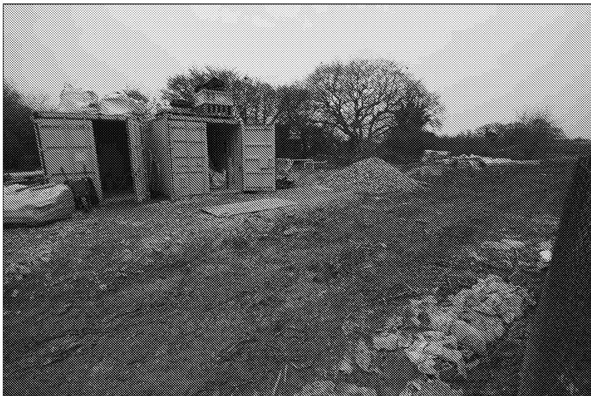
Photo 4: Works area in north east field of Phase 4&5. This area is part fenced. The remaining proposed construction area should be cut per the vegetation method statement and potential reptile and bird habitat mitigation implemented. Any remaining tree protection fencing should also be installed.
