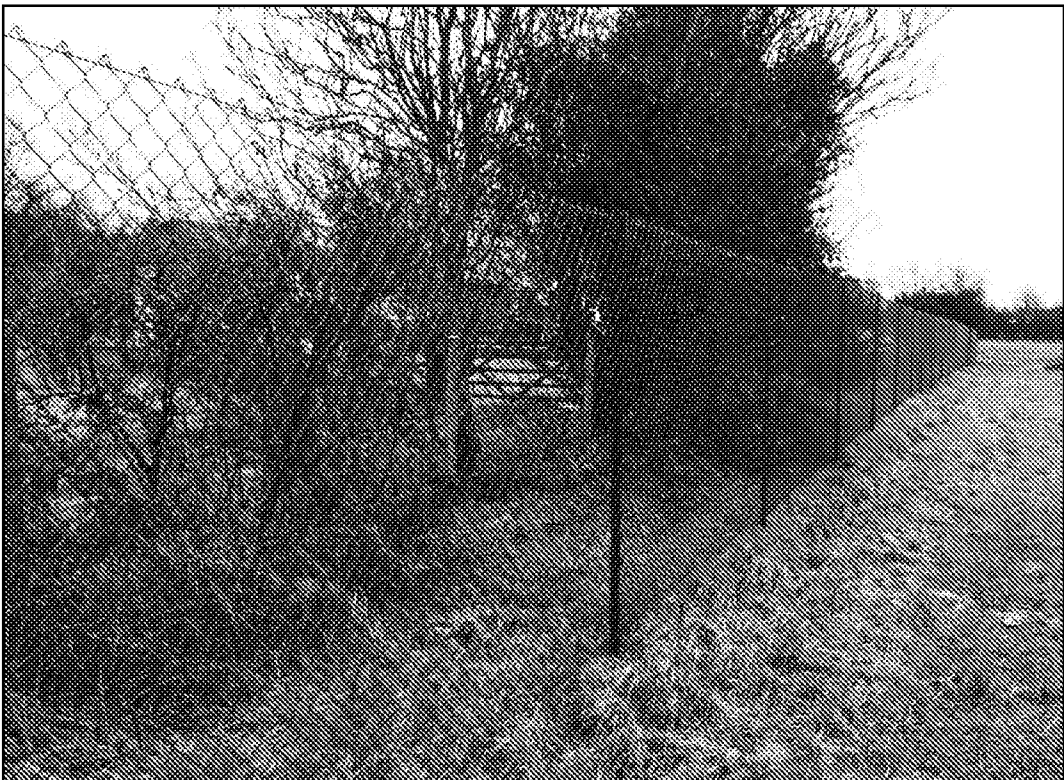
Chain-link on angle-iron uprights
