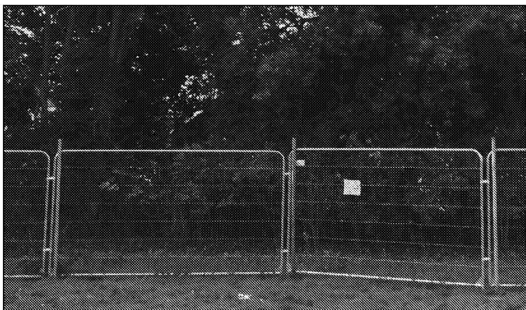
Weld-mesh panels on scaffold uprights
