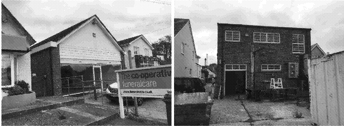
Figure 2 Above Left: Front of Application Site Right: Rear Elevation of 107 Felpham Way Pre-Existing Building
