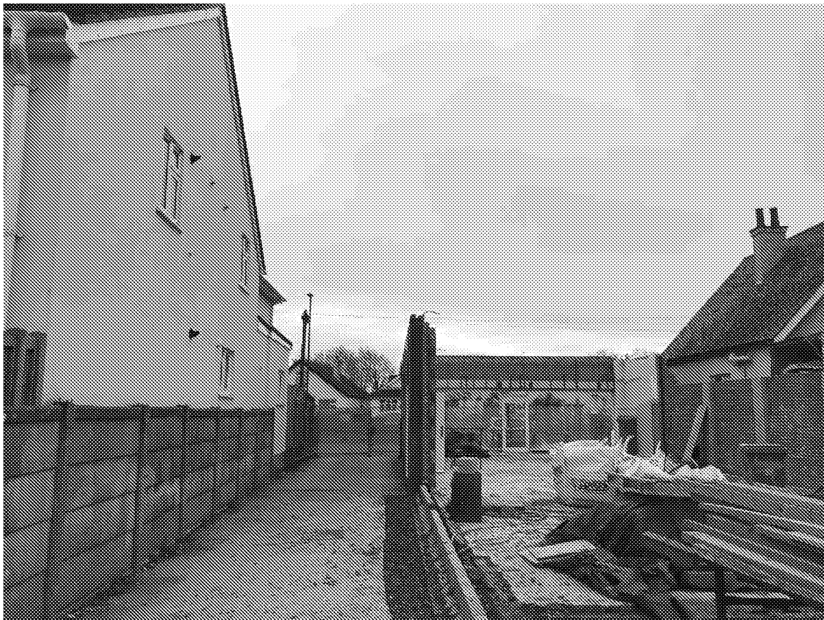
Figure 4 View from Rear of Site towards Felpham Way
