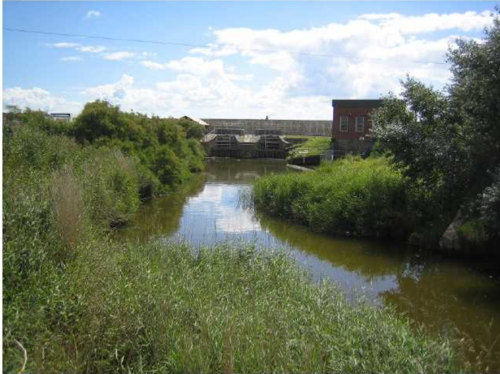
Photograph 9 – Aldingbourne Rife double outfall into the sea and the Felpham Pumping Station to the right
