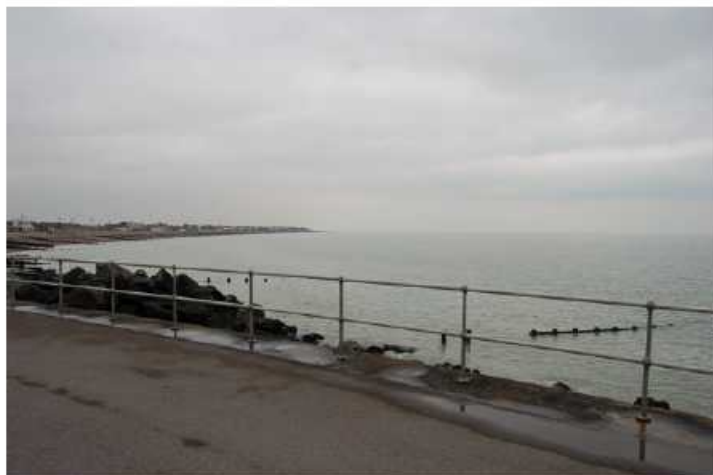
Photograph 5 – Flood defence wall and boulders in front of the site
