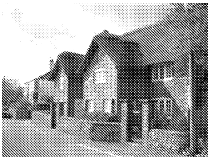
Figure 31 Pear Tree Cottage, Vicarage Lane
