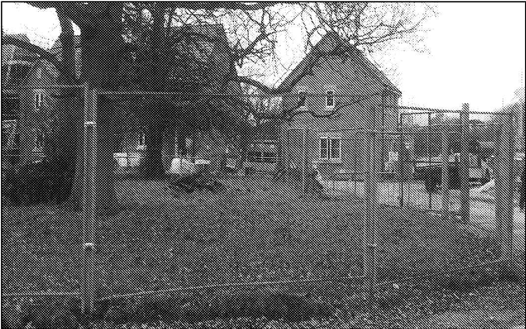
Weld-mesh panels on wooden posts
