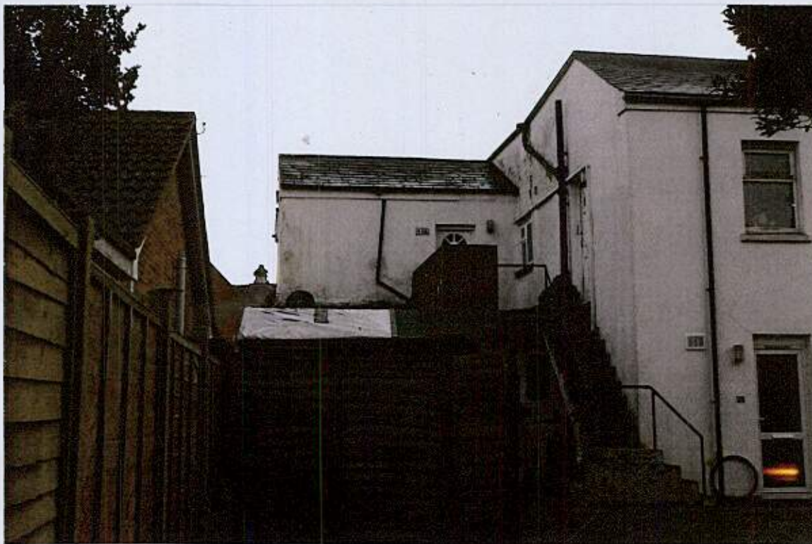
Photo. F - Single storey extension on boundary to be demolished.
