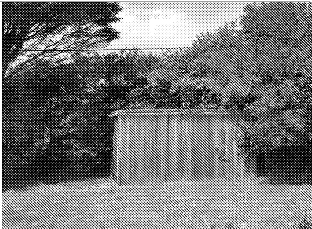
Photo 3: The small shed on the western boundary of the site. Considered to contain negligible bat roost potential.
