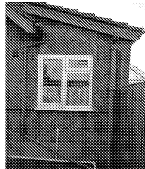
View of side (East) elevation of existing rear extension
