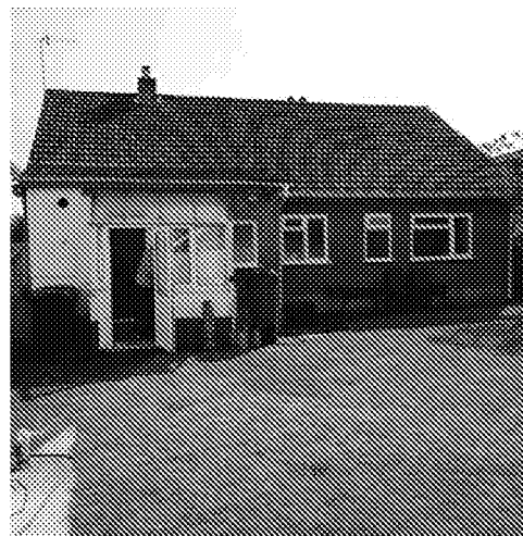
View of the rear of the house from the garden
