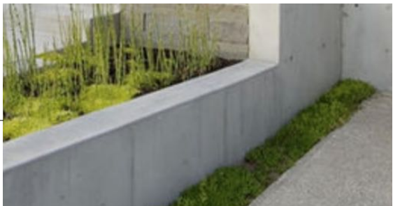
Images of low retaining wall along boundary with Clyde road, natural cast concrete finish.
