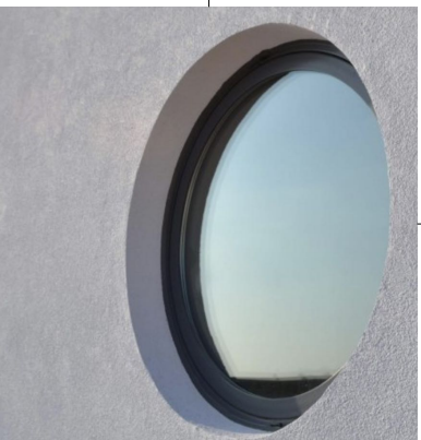
Images of porthole windw, to be finished in PPC RAL 7004
