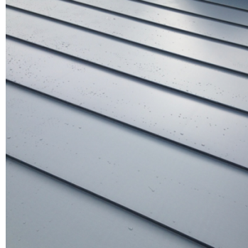
Roof – Standing seam zinc
