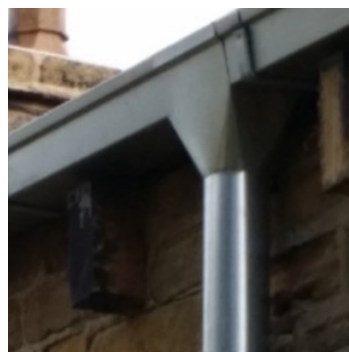
Gutters and downpipes – Galvanised steel – Lindab box gutter
