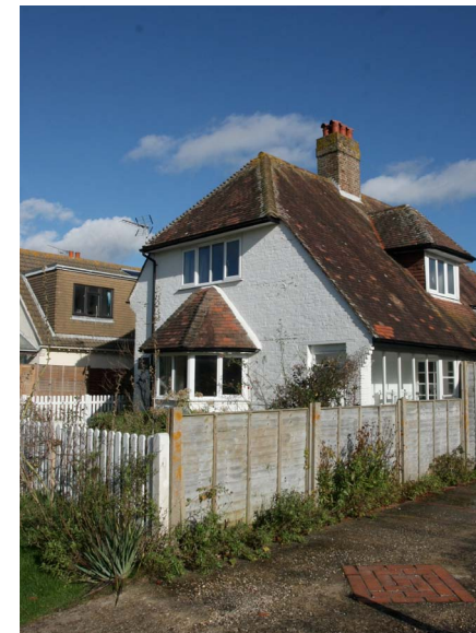
View showing proximity of neighbouring property
