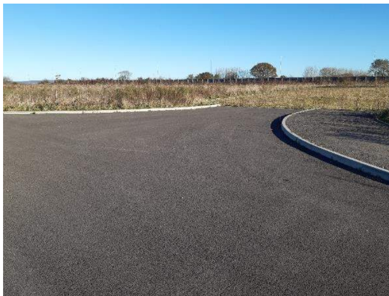
Photograph 2: Access road and pavement
