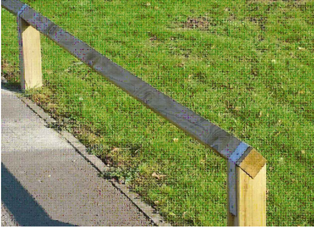
Knee rail fence to site boundary
