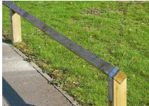
Knee rail fence to site boundary
