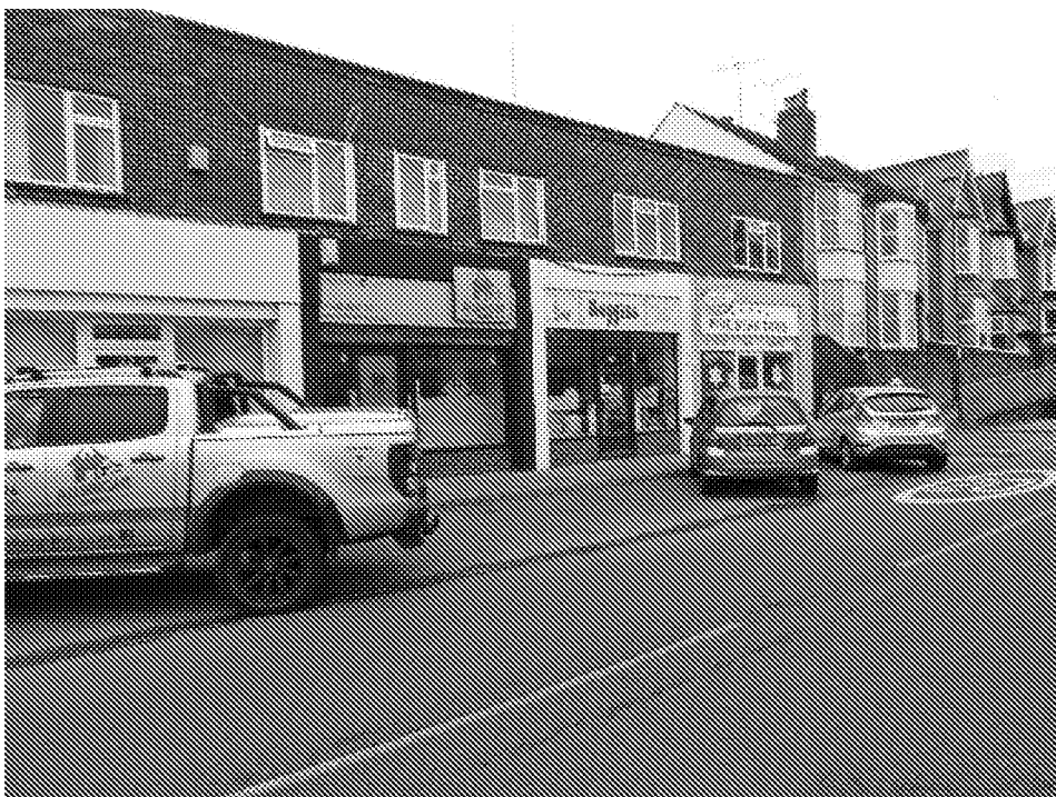
3 – Adjacent retail premises
