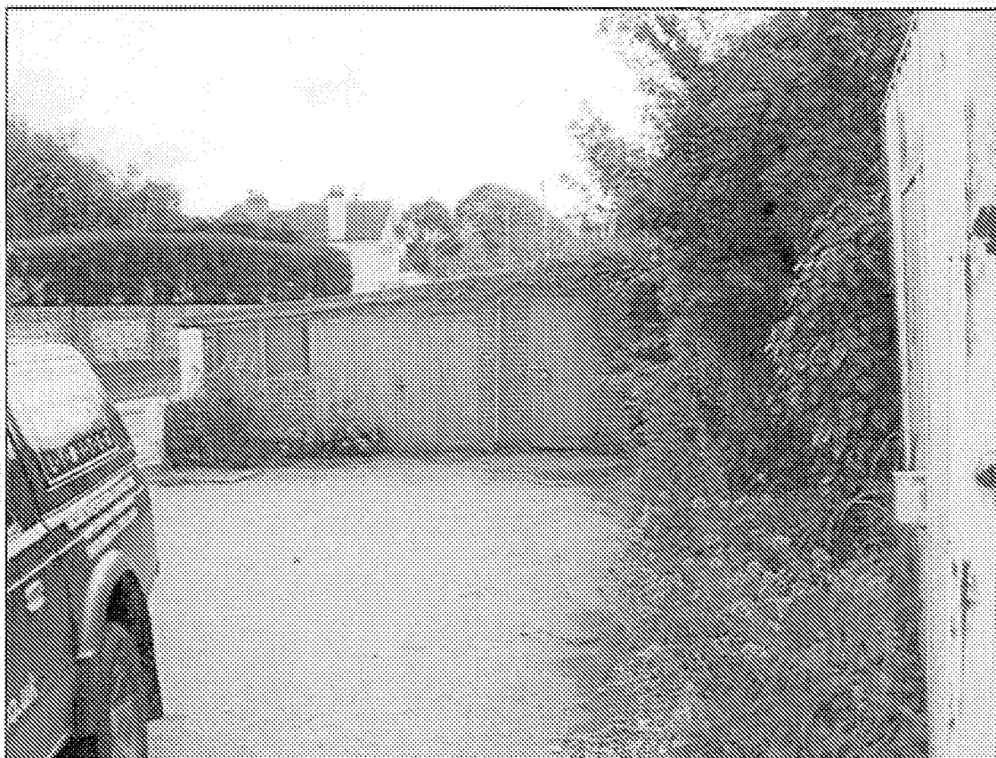
Photo 1 - Showing garage (North East corner of the Site).
