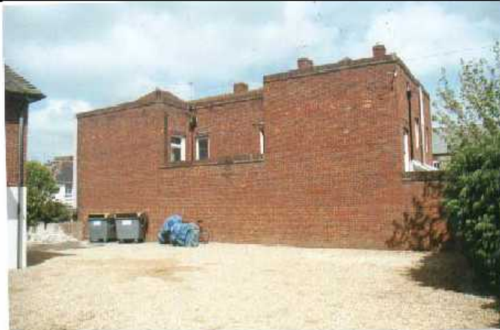
View from South – Richmond Villas
