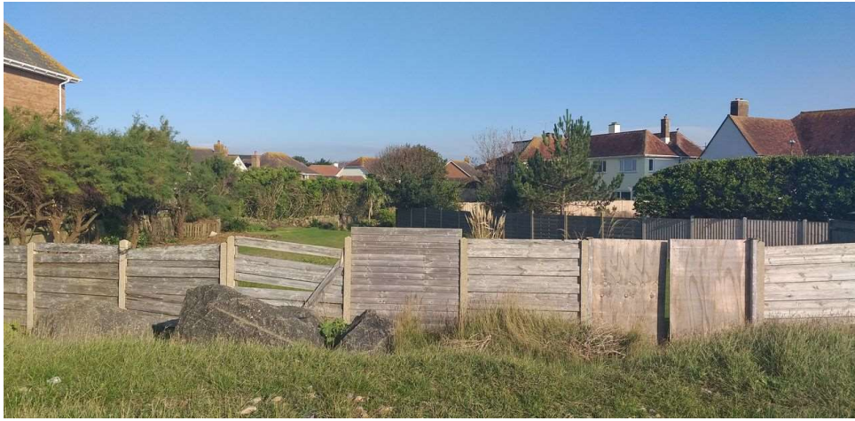
Promenade grass bund view north
