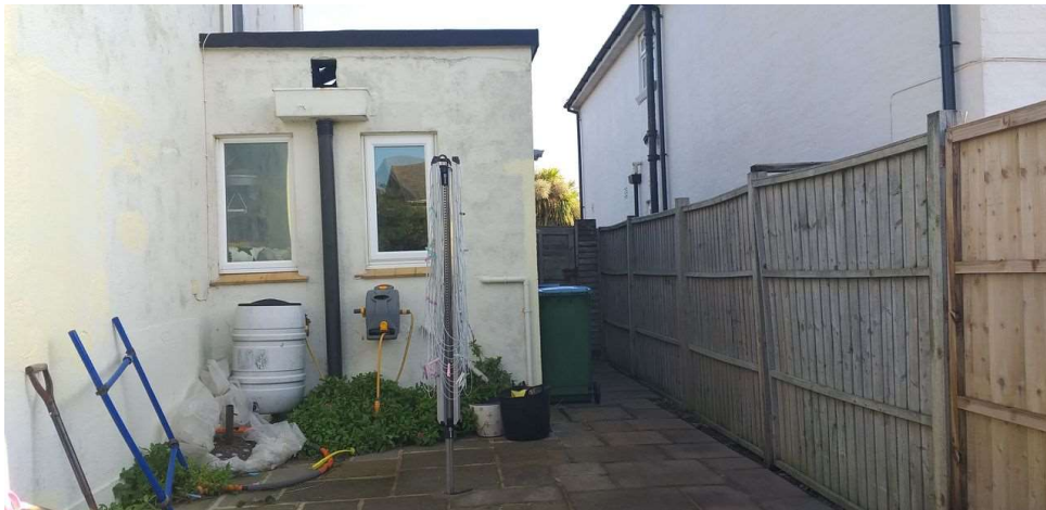
West face of utility room to be removed, 3.8m between retained house wall and fence
