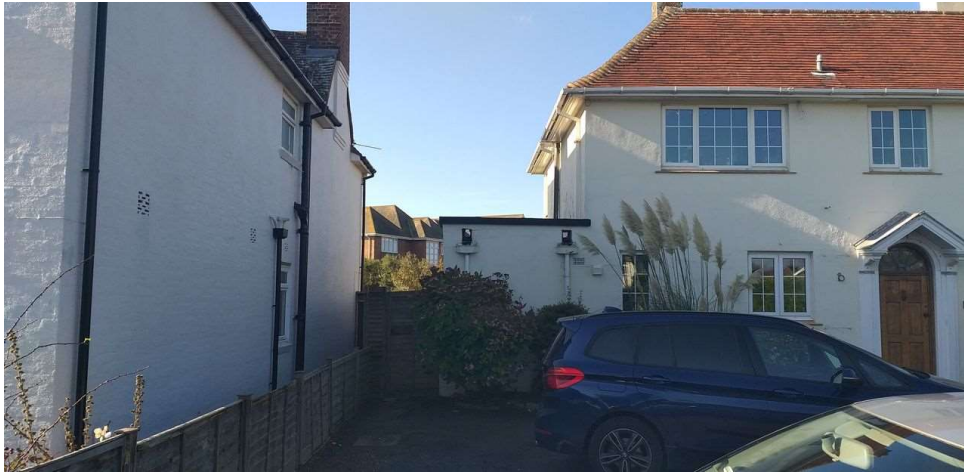
East face, line of new drive with removal of flat roof utility room
