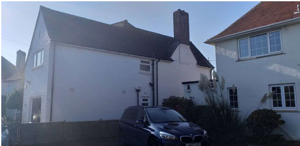
North side of No 5 The Loop
