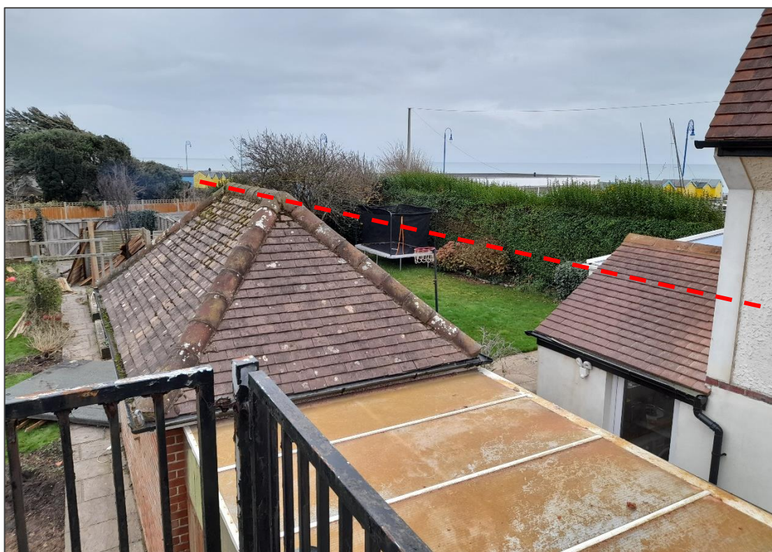
Plate III : View from existing rear (east) roof terrace toward south boundary Dashed red line indicates the approx. ridge height of the proposed roof over the garage and Leisure suite. This is felt to provide enhanced privacy for both 15 and 17 Blakes road.
