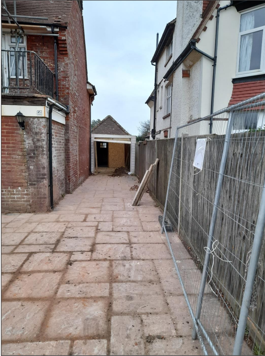
Plate I : View of South Boundary adjacent 17 Blakes Road
